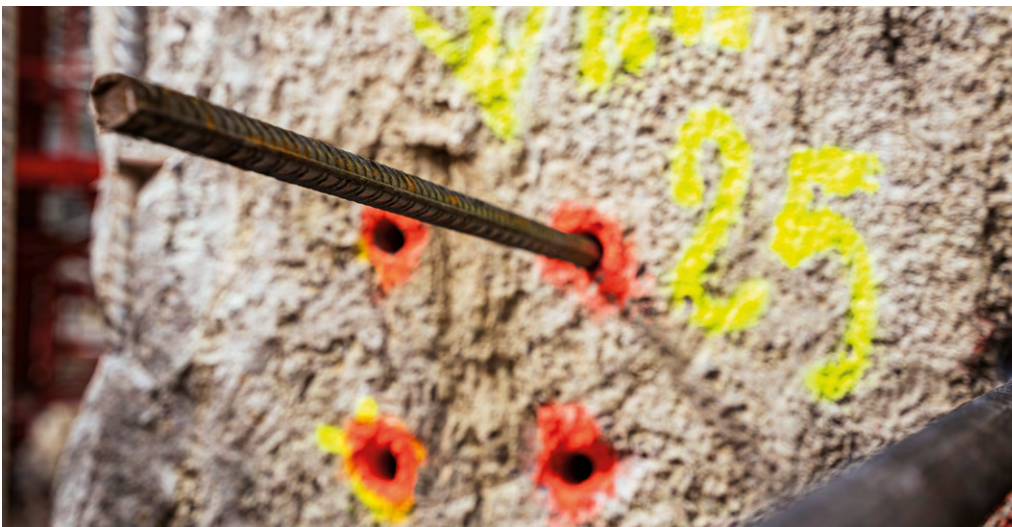
A post-installed rebar on a construction site.
